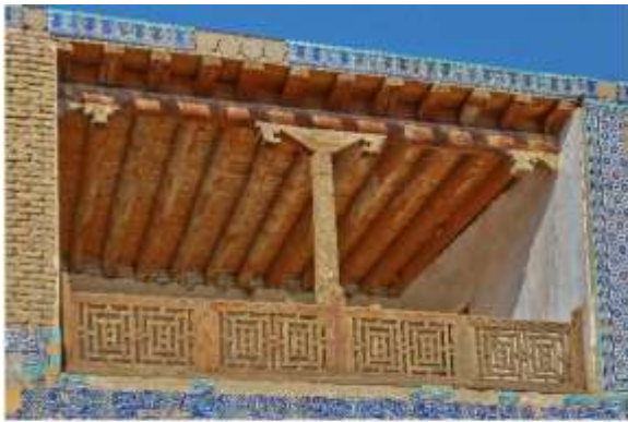
Figure 1. Traditional Ayvan. Principles of deep shading and wooden latticework in Khiva architecture.
