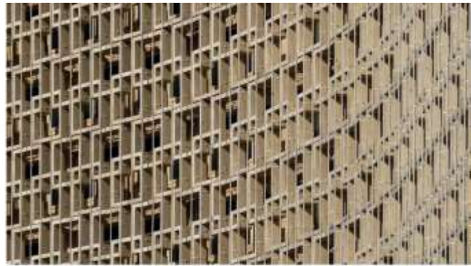
Figure 2. Three-dimensional geometric screen, Modular grid system of the "Uzbekistan" Hotel facade in Tashkent.
